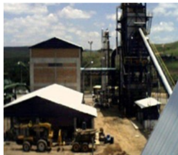
Piratini-Wood Chips Power Plant, Brazil 2004 | €25mm
