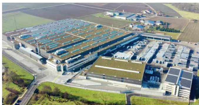
Plant 3 in Cleebronn
